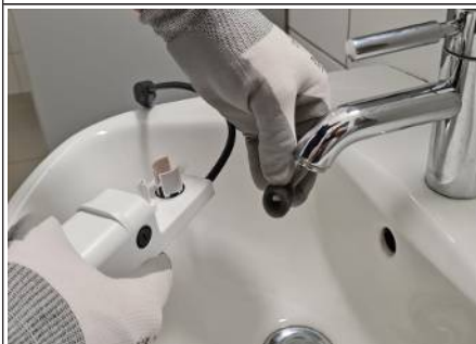
Fig. 20: Cleaning the dirt filter
