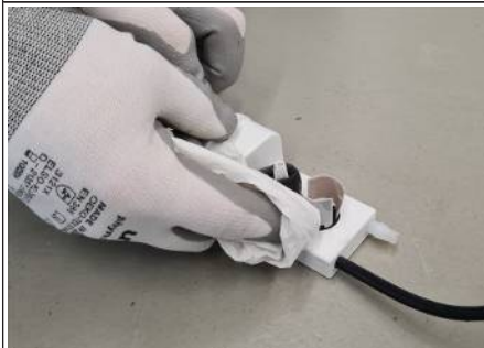
Fig. 19: Cleaning the condensate pump
